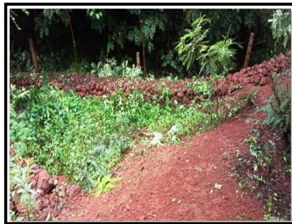
(View of Retaining wall around OB Dump)
